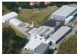
Werk Ledec nad Sázavou Czech Republic
