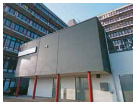
The 450 m 2 "New Data Centre" at University of Siegen
